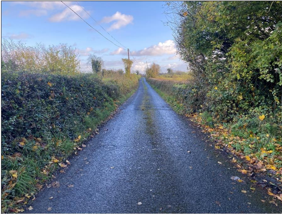
Plate 6-29 Route for grid connection underground cabling on road crossing at Clonmore river bridge located at the south east of the Site.
