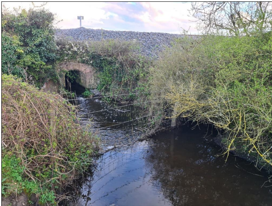
Plate 6-31 View of the proposed clearspan bridge location with an existing tunnel within the railway located at the southeast of the Site near where the proposed grid connection underground cabling access road will pass by.
